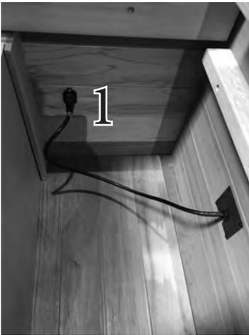
4. From the hole in the floor, take the short heater cable labeled "HEATER" and plug into power supply.
