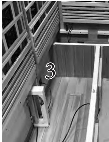
5. From the hole in the floor, take the long heater cable and plug into the bench heater connector.
