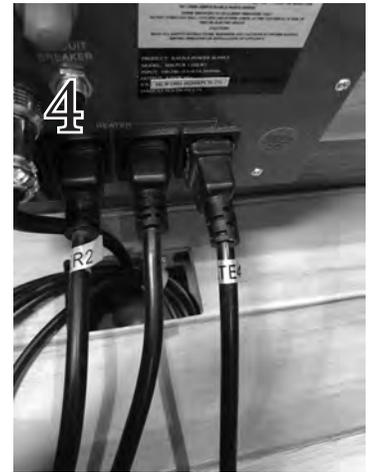
2. Plug the cable coming out of the bench heater into any of the 4 "HEATER" sockets on the power supply mounted in the back panel. This cable is not marked.
