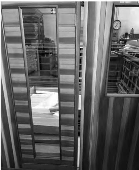
3. Take the front large panel with glass door and place on base. Be careful to not allow the door to swing and accidentally break the glass.
